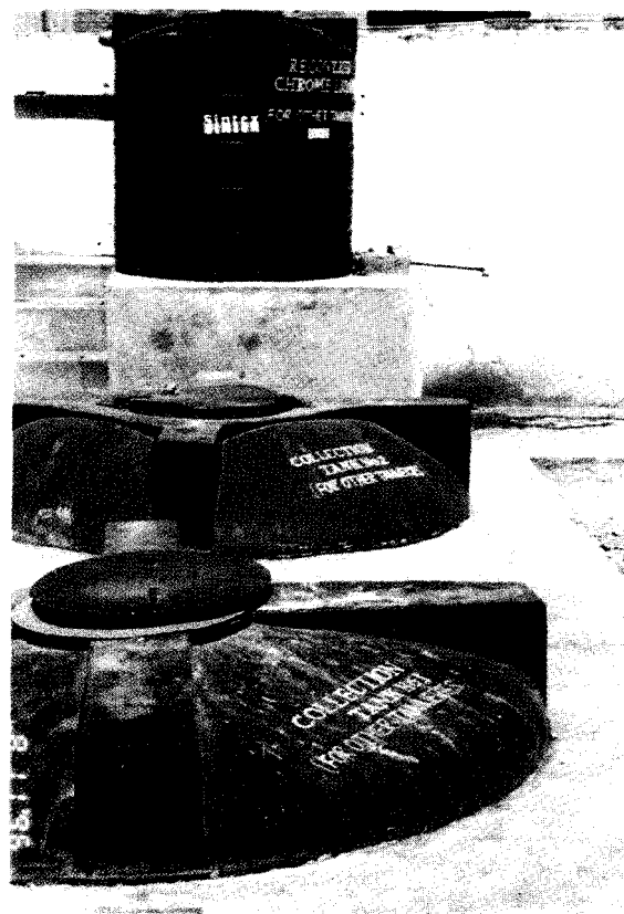
Collection tanks for common chrome recovery system
